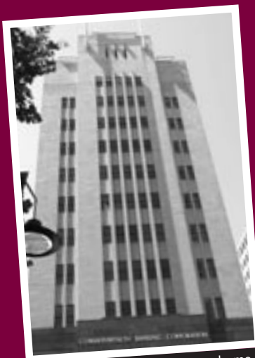
225 Bourke Street – our new home.
